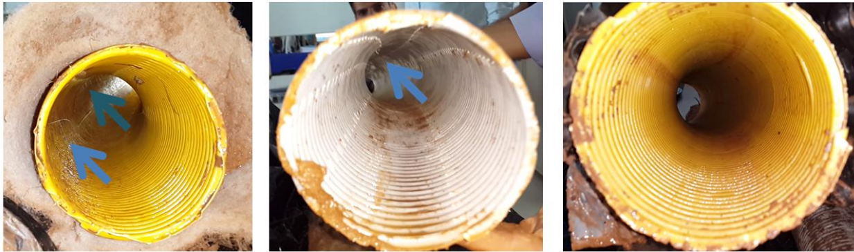
Figure 7. Visual inspection for root growth after excavation of the drain pipes with a geotextile (left), no envelope (middle) and Hydroluis® combination (right).
